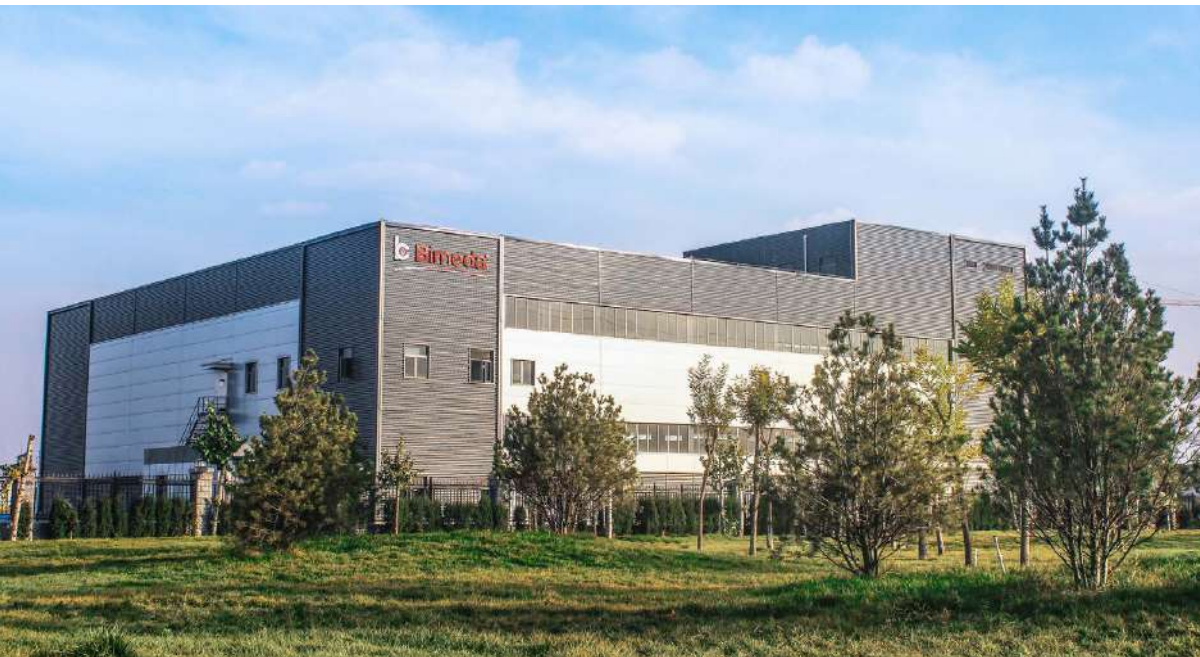
Bimeda Facility in Shijiazhuang, Hebei, China
